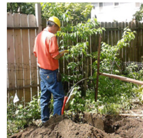
GPS new underground secondary line
